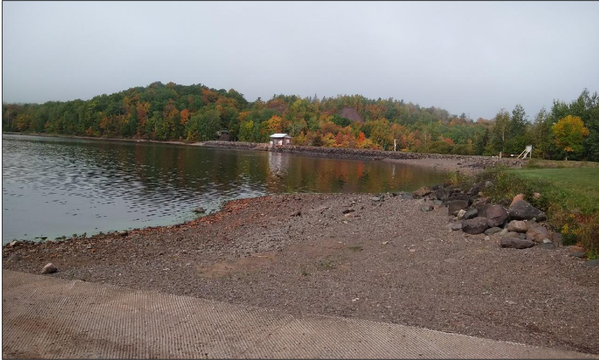
Figure 4.9.1-2: View of Project Dam
